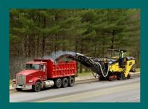
Mill and Fill is a structural pavement treatment that involves the removal of the existing surface layer with a milling machine and the replacement of the milled location with new asphalt. This restores and strengthens a road's surface layer by replacing the pavement's top wearing course.
