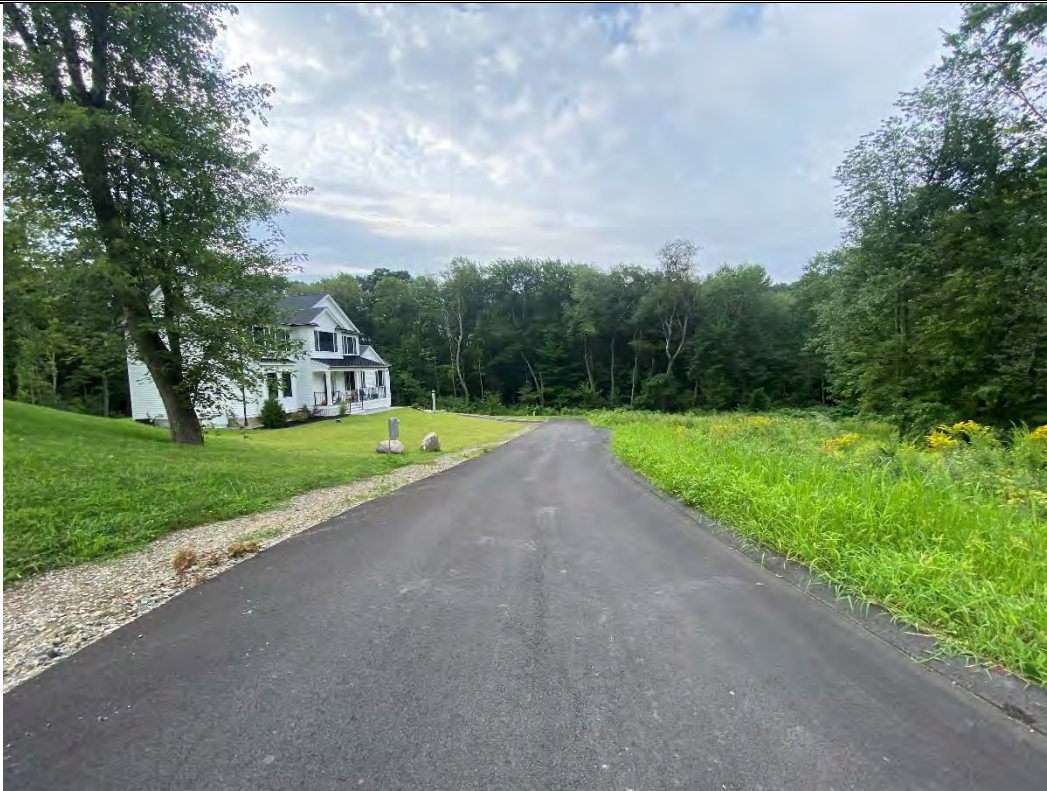
Figure 3 – Overview along the Extension. Photo taken facing south.
