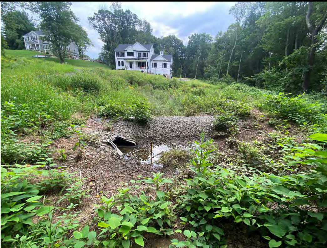
Figure 6 – Overview of the Infiltration Basin. Photo taken facing east.
