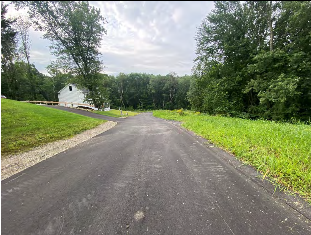
Figure 2 – Overview along the Extension. Photo taken facing south.
