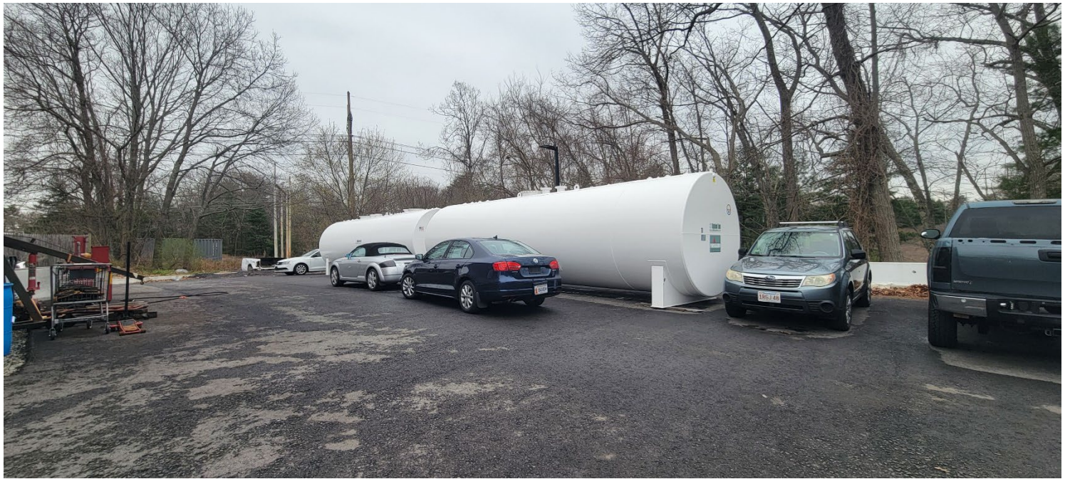
Figure 6 – Stockpiled proposed gas tanks to be placed in vault, south of existing garage. Photo taken facing southeast.
