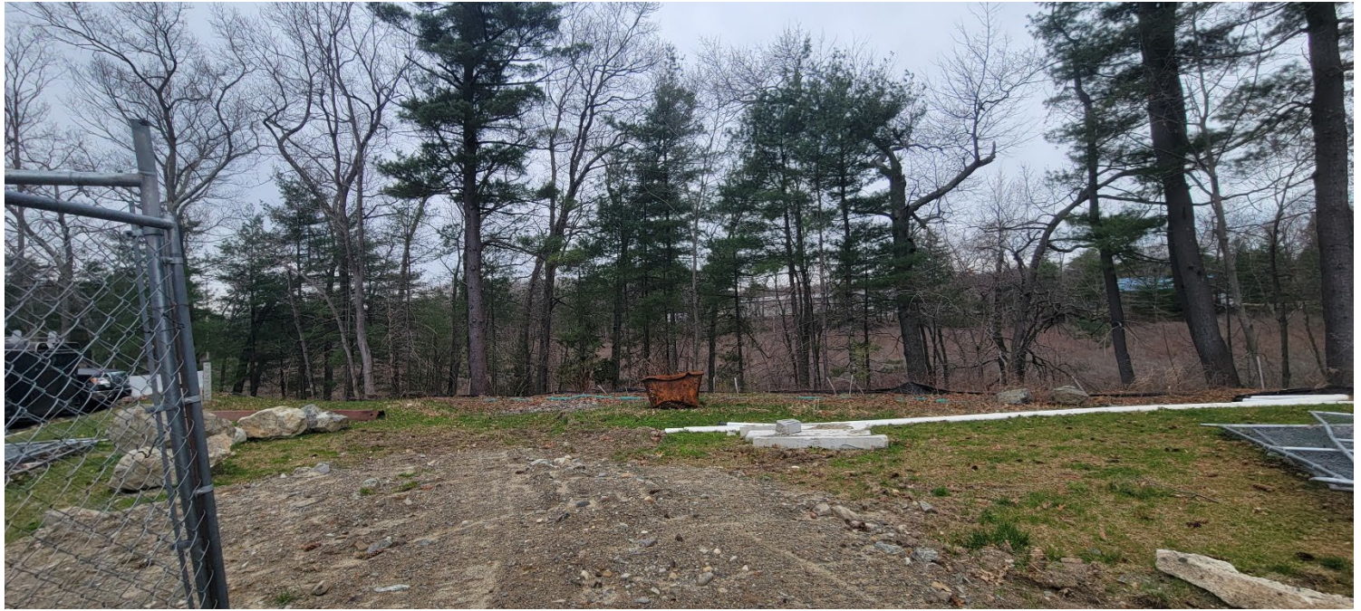
Figure 5 – Sagging silt fence located near the southwestern site limit. Photo taken facing south.
