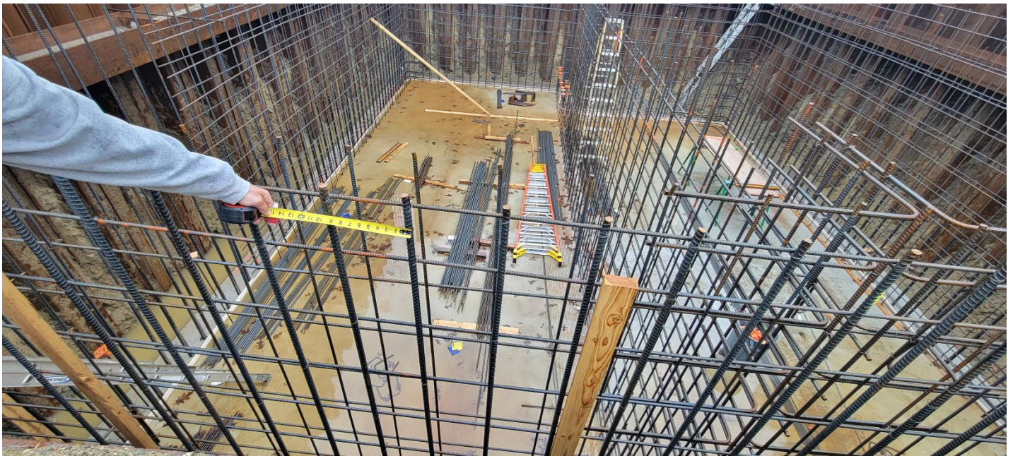
Figure 2 – Example measurement of the “exterior” vertical bar (#7) spacing. Photo taken facing south.
