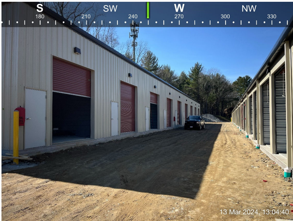
Photo #8: Looking between Buildings #3 & #4. Stabilized, compacted gravel in place.
