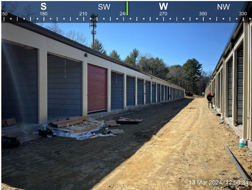
Photo #7: Looking between Buildings #2 & #3. Stabilized, compacted gravel in place.
