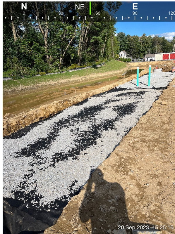
Photo #13: Photo taken on 9/20/2023 prior to backfill of Chamber System #1.
