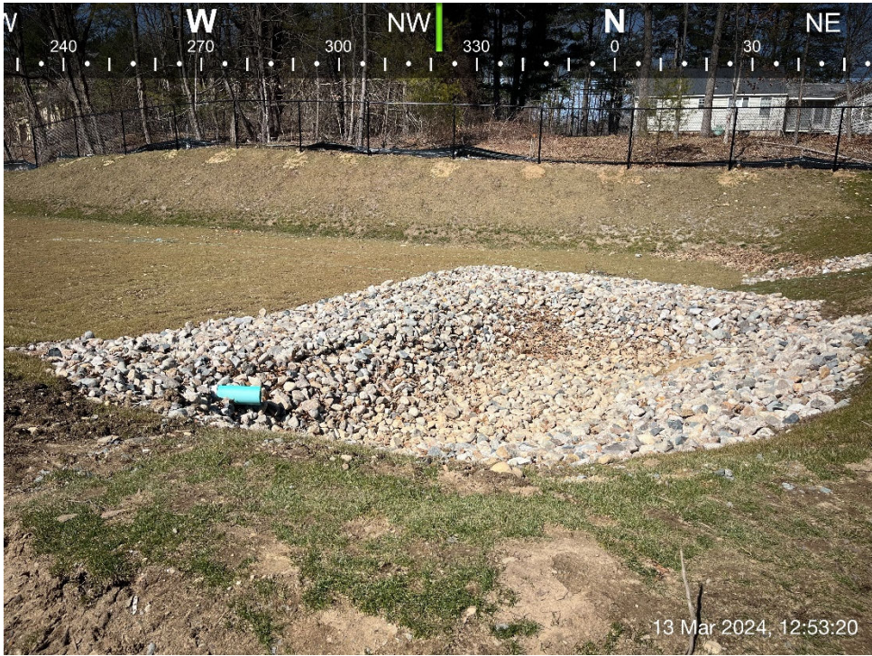
Photo #4: Forebay #1. Stone in place and showing signs of good operation.
