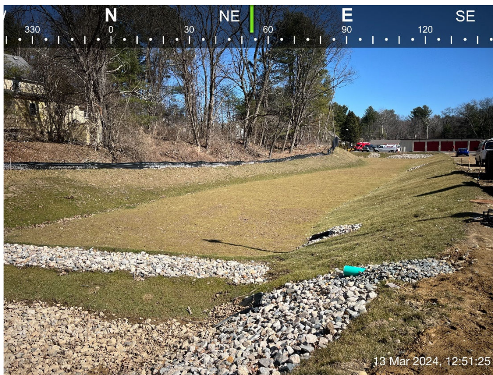
Photo #2: Infiltration Basin #2. Good percentage of vegetation growth via seeding last summer.
