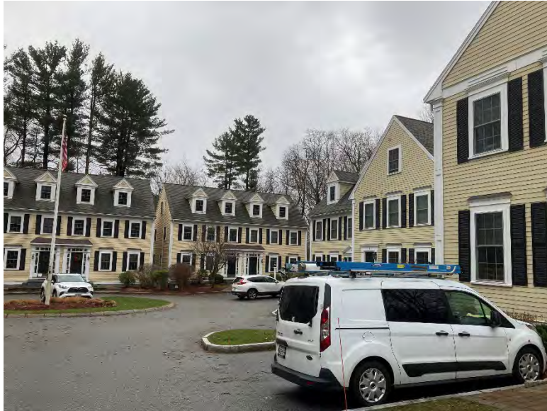
Multifamily Amesbury RKG Associates
