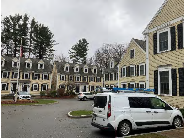
Multifamily Amesbury RKG Associates
