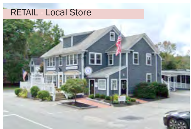
Fg 45. Boxford Community Store & Kitchen, Boxford, MA
