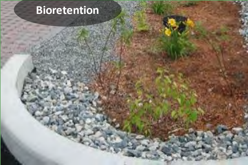
Bioswale Stormwater Treatment
