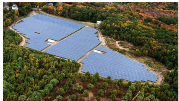
Fig 21. North Brookfield 2.5MW Solar Project (© Mass Electric Construction Company)
