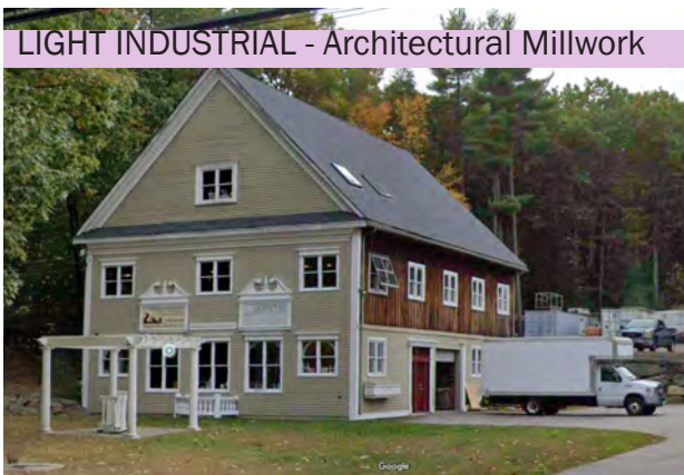
Fig 38. Architectural Elements, Inc., Boxborough, MA
