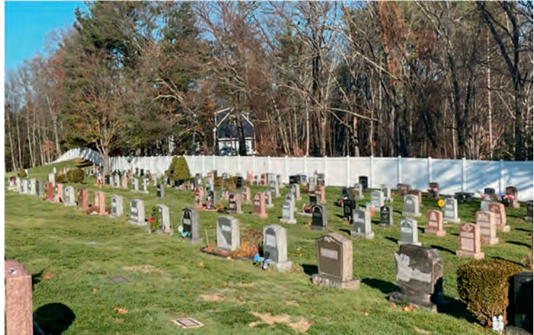
Pictured above: Riverview Cemetery looking east at the new vinyl fence installed.
