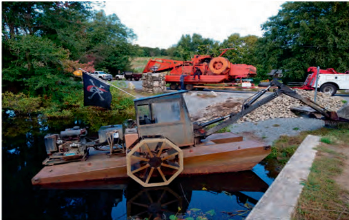
Photos from the approved FY2021 Weed Removal Project completed in October 2021
