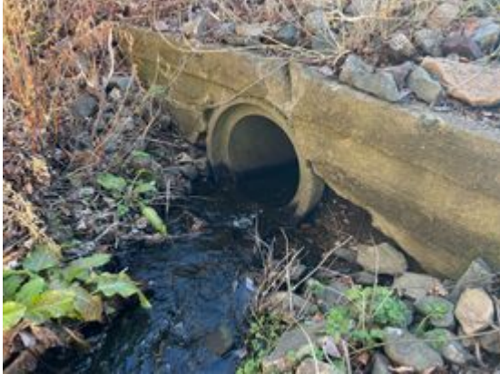
Photo 1: Upstream Photo of Culvert / Dam
