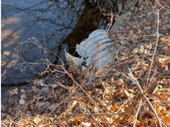
Photo 1: Upstream Photo of Culvert / Dam
