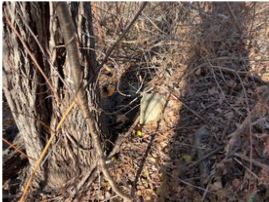
Photo 3: Downstream Photo of Culvert / Dam
