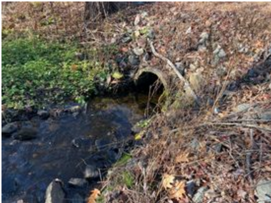
Photo 3: Downstream Photo of Culvert / Dam
