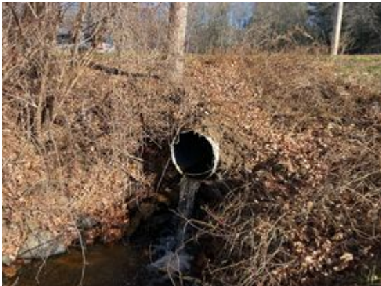
Photo 3: Downstream Photo of Culvert / Dam
