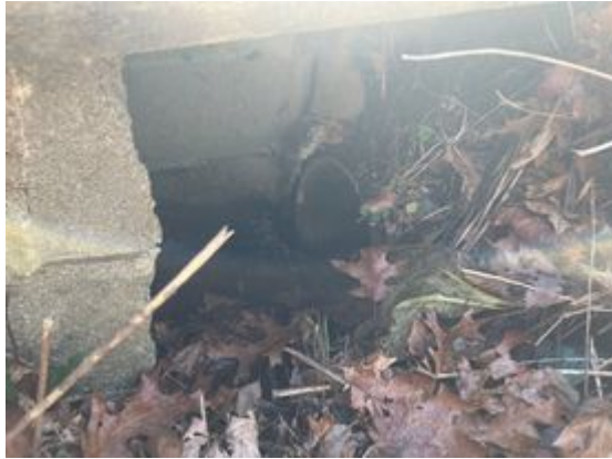
Photo 1: Upstream Photo of Culvert / Dam
